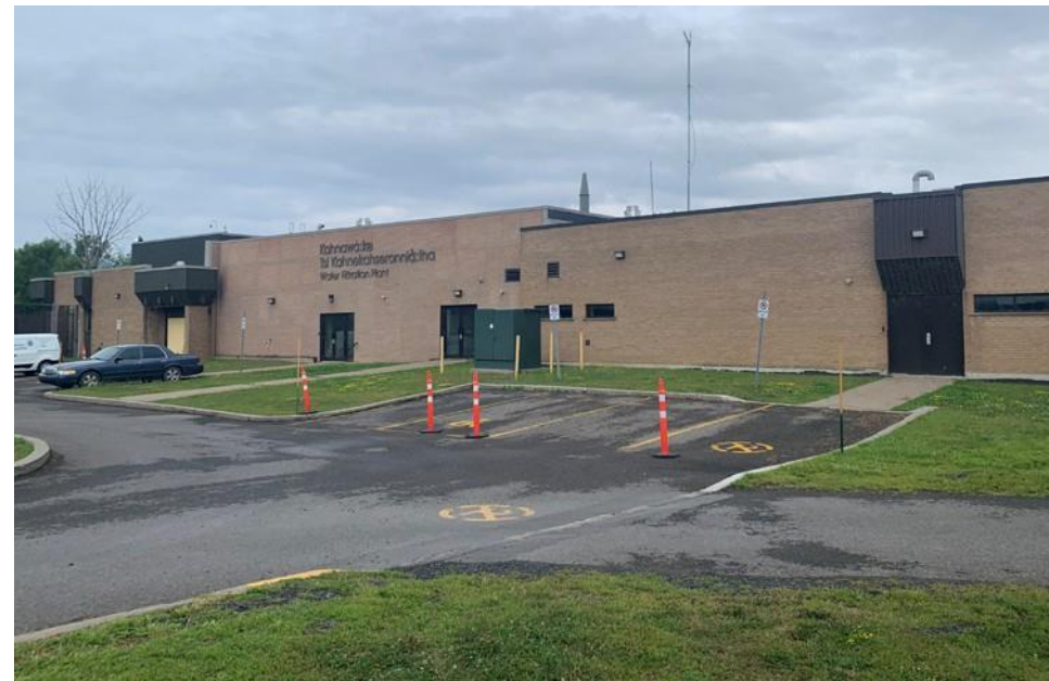
Photo of the Kahnawà:ke Water Filtration Plant
