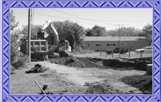
Capital crew doing road work on River Road
