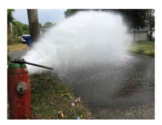
Unidirectional flushing is the process of cleaning the water system by flowing water in one direction through the water mains. This is accomplished by closing specified valves and by flushing strategically located fire hydrants.
